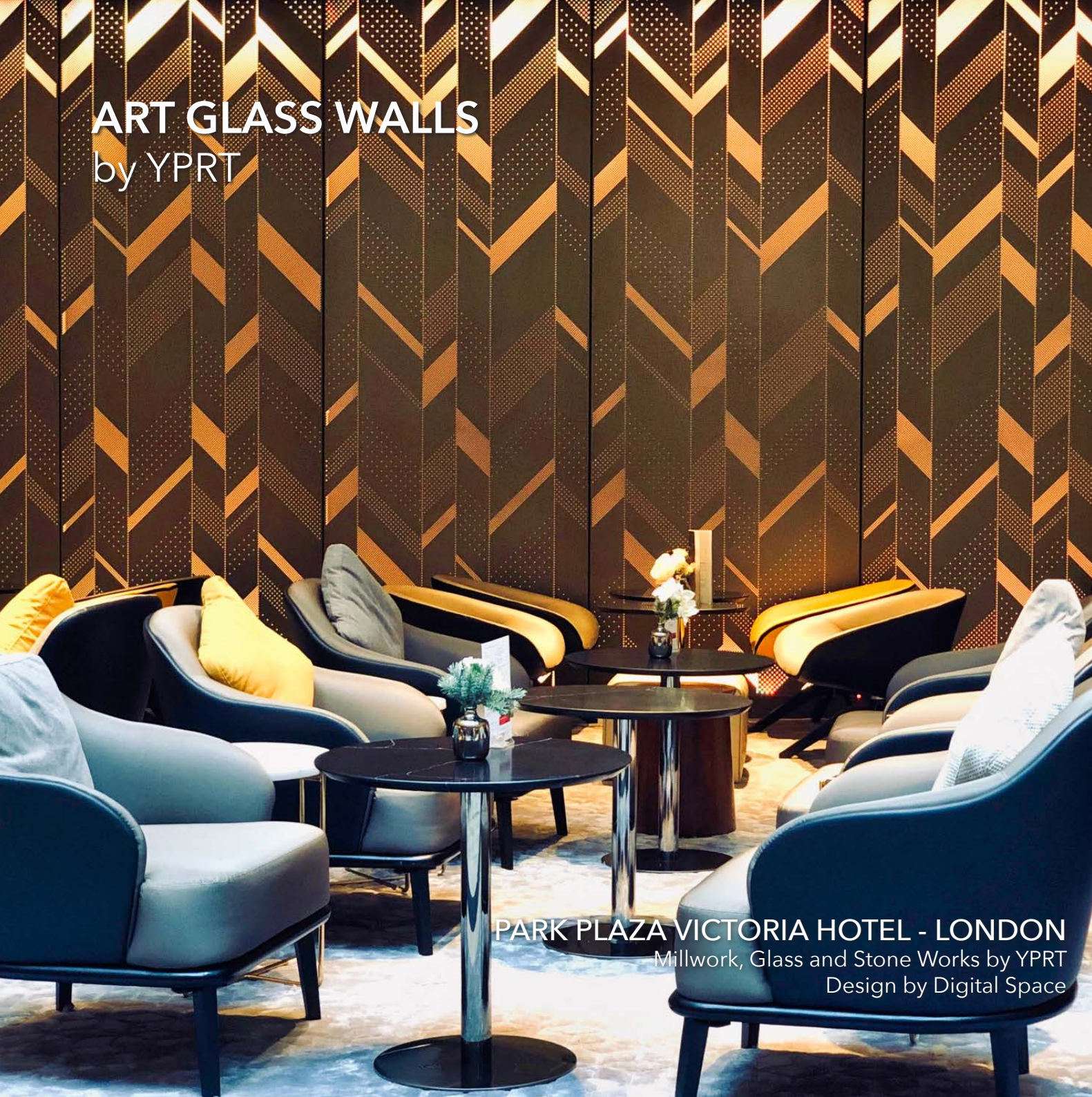
Park Plaza Victoria Hotel - London Digital Printed Tempered Glass with MDF support Powder Coated Metal Frame
