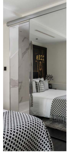
Sliding Mirror Door Clear Mirror on MDF Chrome Plated Metal Outer Frame Stainless Steel Handle
