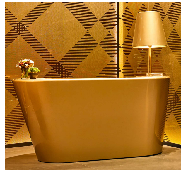
Victoria Hotel - Amsterdam Glossy Painted Fiberglass Unit Steel Interior Structure Painted MDF Interior Cabinets Tempered Glass Counter Top
